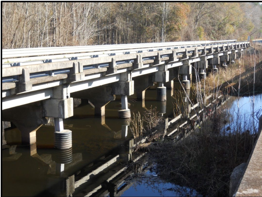
Figure K.2: US 301 SB Bridge
