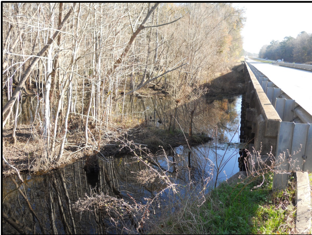
Figure K.6: Upstream Side of US 301 Bridge
