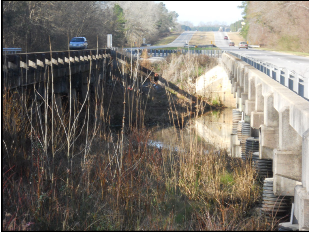
Figure K.1: Area Between Upstream and Downstream US 301 Bridges
