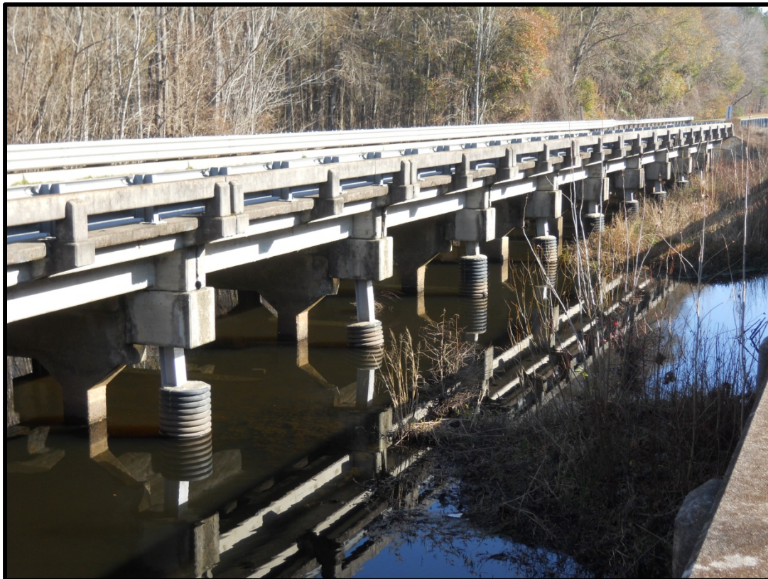
Figure K.2: US 301 SB Bridge
