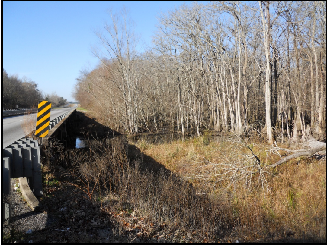
Figure K.3: Upstream Side of US 301 SB Bridge
